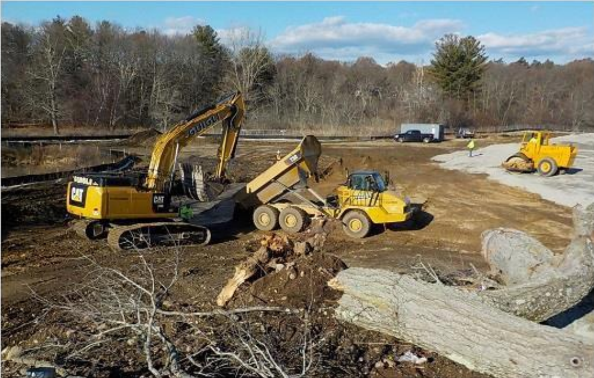
Looking North at Unsuitable Soil Removal East of Pond 2017.12.07
