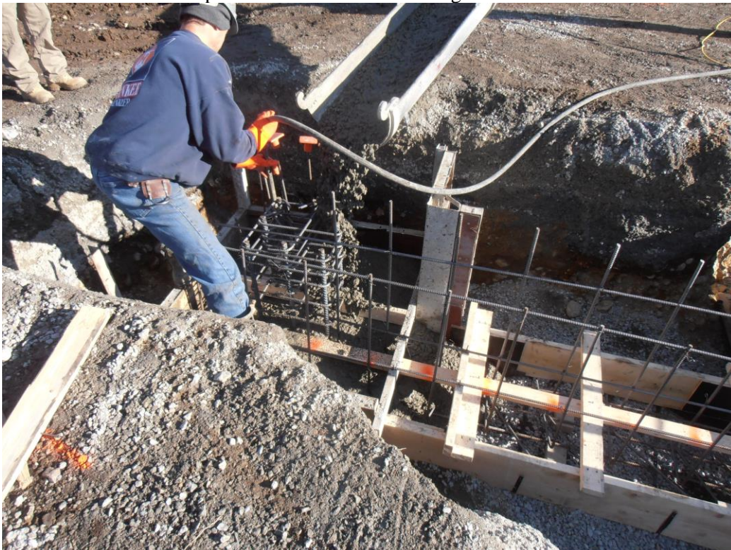
First Concrete pour – NW Corner of Building – 12/20/2017
